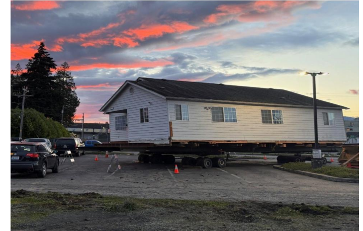
Figure 7: Building Deconstruction Washington, United States.
