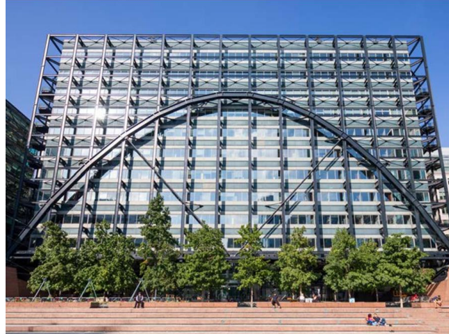
Figure 6: The Exchange House London, United Kingdom
