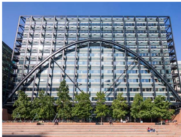
Figure 10. The Exchange House London during Renovation (WBCSD, 2021)
