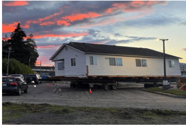
Figure 8. Relocating a Building to a new lot through Deconstruction at Port Angeles (GLY Construction).
