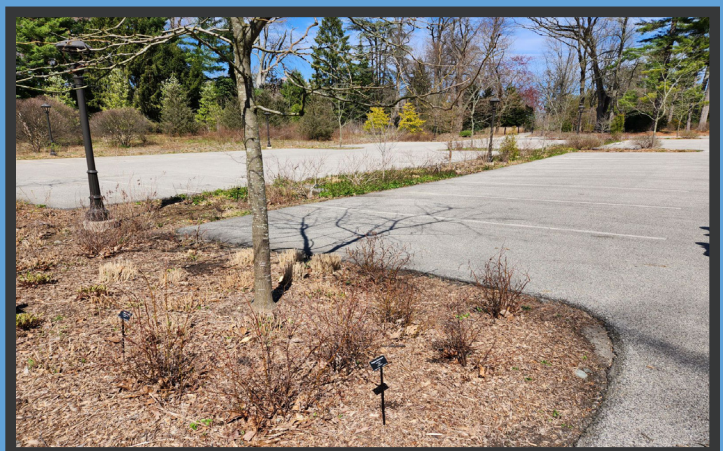
Bioswales are landscape features that collect polluted stormwater runoff, soak it into the ground, and filter out pollution.
