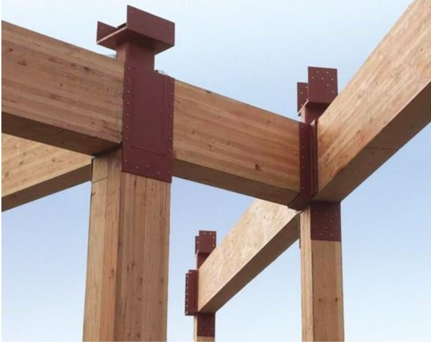
Figure 2.1: Steel connectors are located at each connection point.(Bullitt Center, Seattle, WA, USA; 2011)
