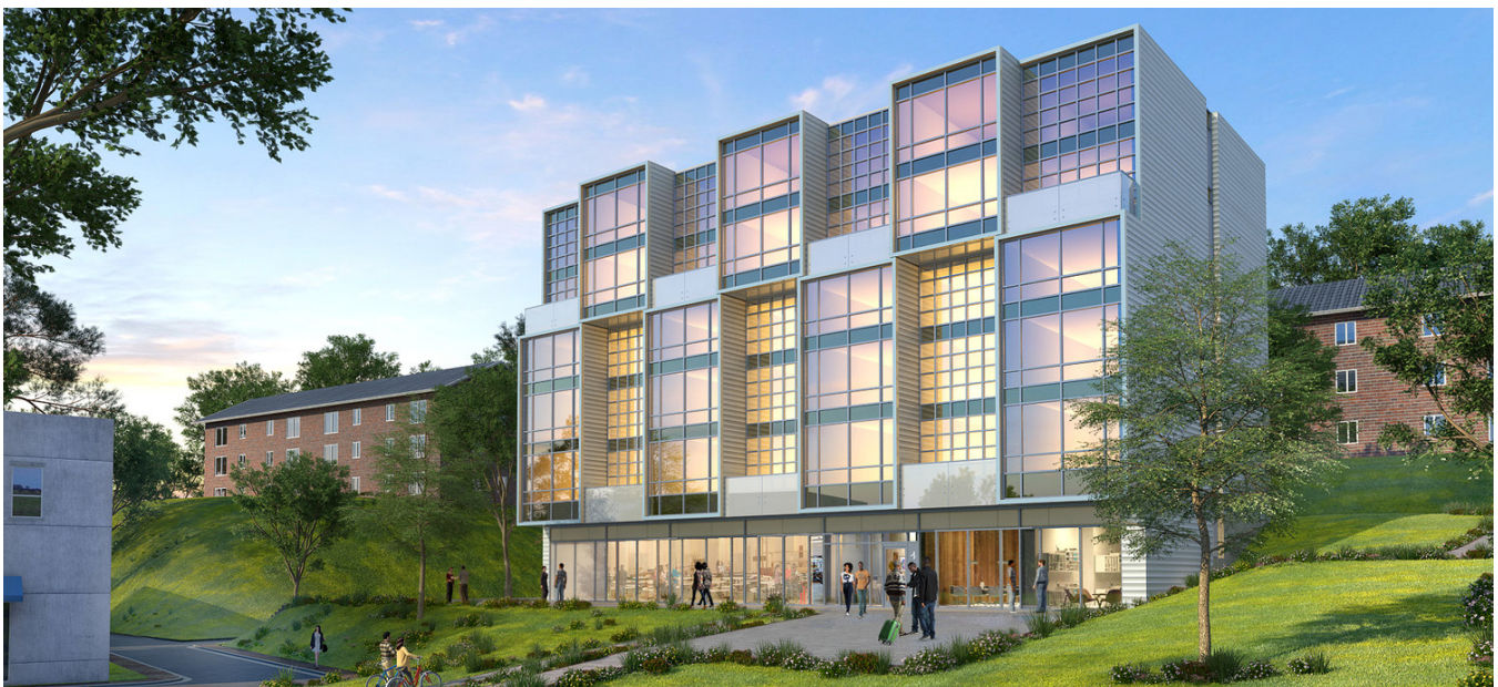
Figure 21: Exterior view with reduced ground floor and residential floor setback removed; Source: CS-A Final Presentation Document
