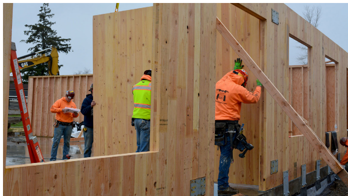
Wood Rich Classroom: Maple Elementary School - Seattle, WA. CLT construction exposed in classroom.
